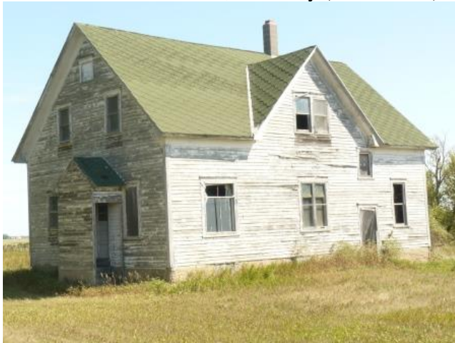
North farmhouse at Oak Lake prior to demolition.
