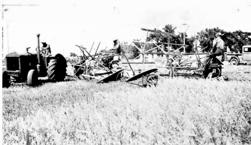
Fig. 4. Making a turn with the two-binder hitch. Notice the square corner.
