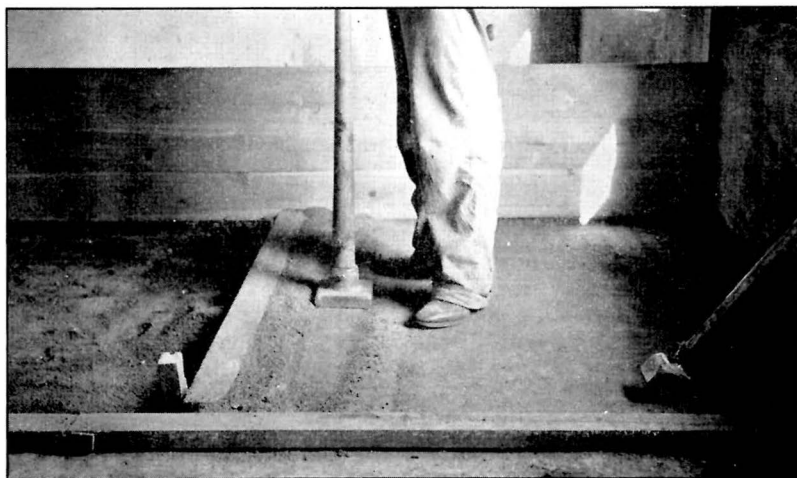
FIG. 9. FINISHING THE SOIL-CEMENT FLOOR.
