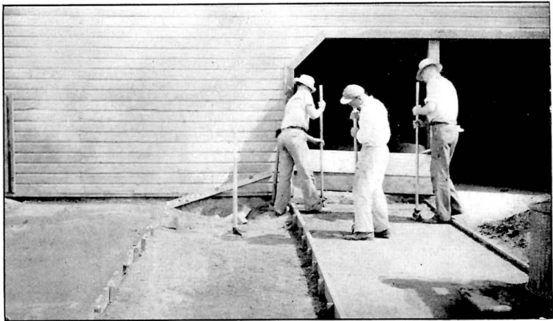
FIG. 7. BUILDING A SOIL-CEMENT FLOOR.
