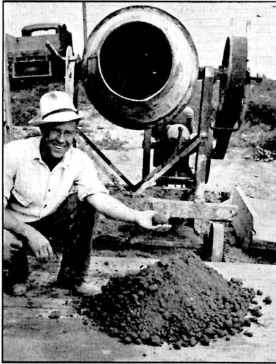
FIG. 5. USING A CONCRETE MIXER FOR THE BASE COURSE.
