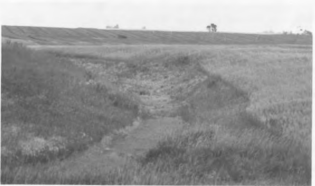
Fig. 6. Typical surface ditch commonly used for wetland drainage in northeastern North Dakota.
