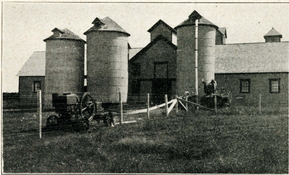
North view of South Dakota State College dairy barn showing two stave silos and one re-enforced concrete silo
