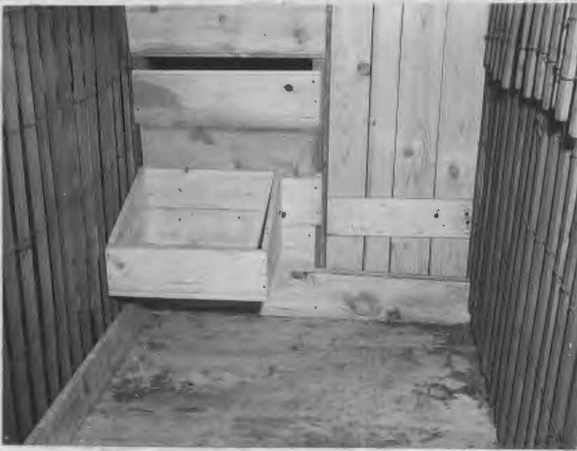
Figure III End view of antelope feeding pen showing feed box and board floor.
