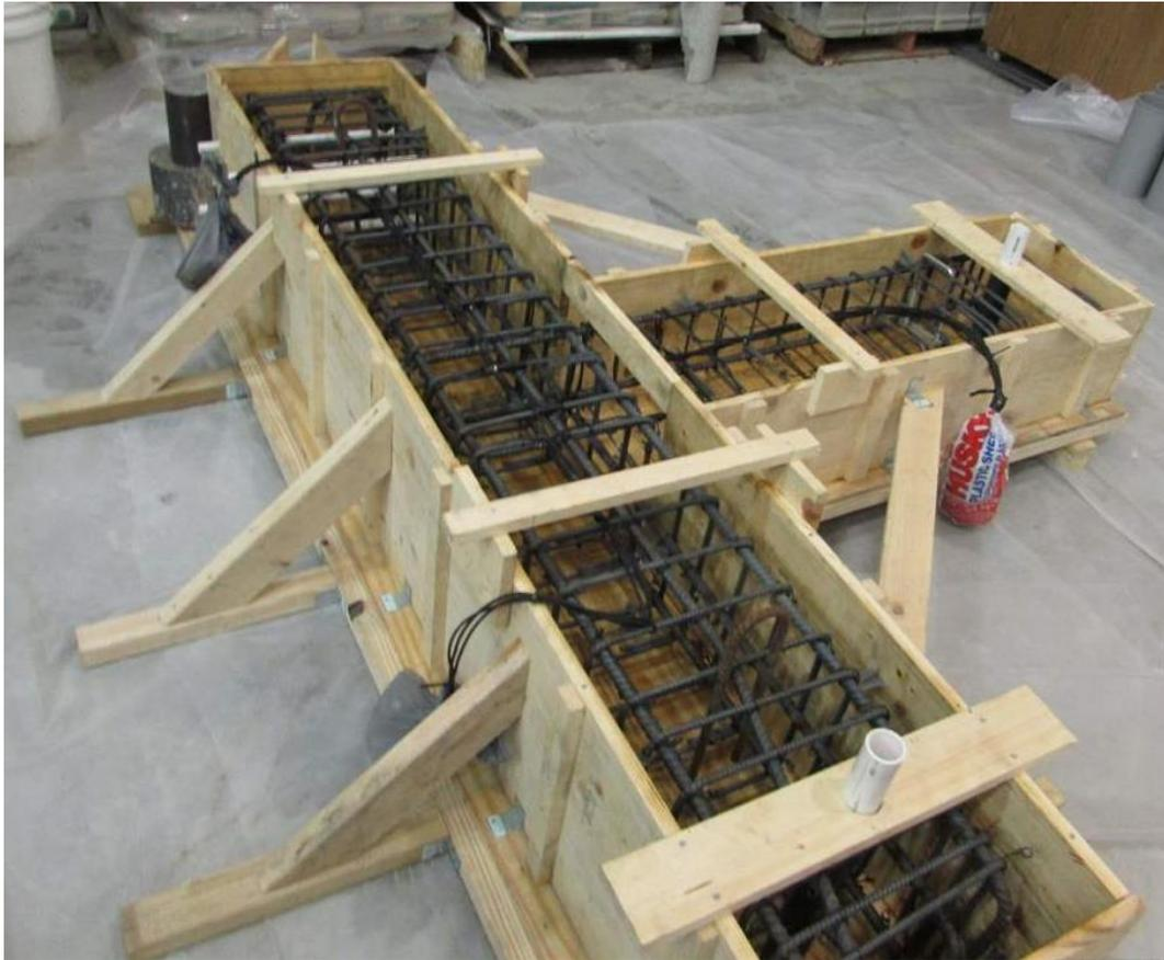
Figure 4-16. Steel cage and formwork
