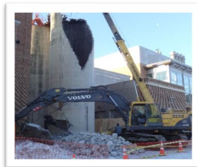
Photo 2: Coal silo demolition.
