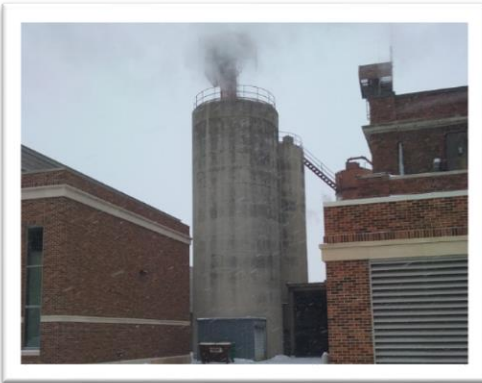
Photo 1: Coal silos prior to demolition.
