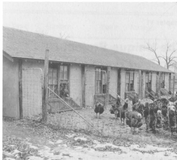
Figure 3. The last of the Rammed Earth Poultry Houses to be built by the Agricultural Engineers.
