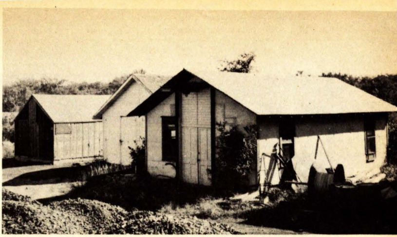
Salt House and Storage Sheds
