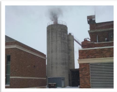
Photo 1: Coal silos prior to demolition.
