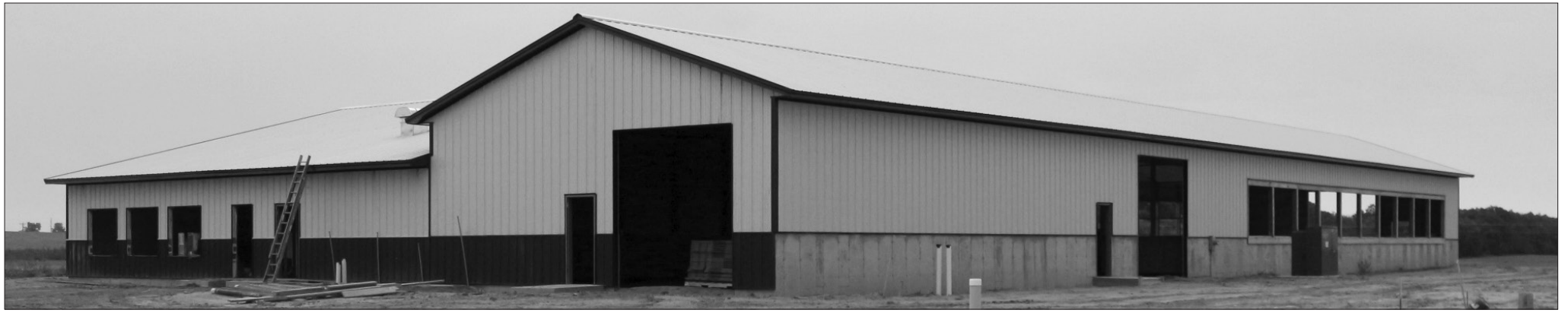
This building will house the classroom, office space, labs, working area and multi-purpose area at the new cow/calf unit.
