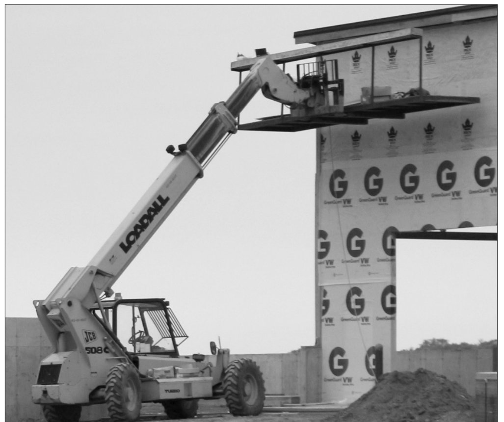
A telehandler hoists building materials and workers at the site of the new cow/calf facilities.
