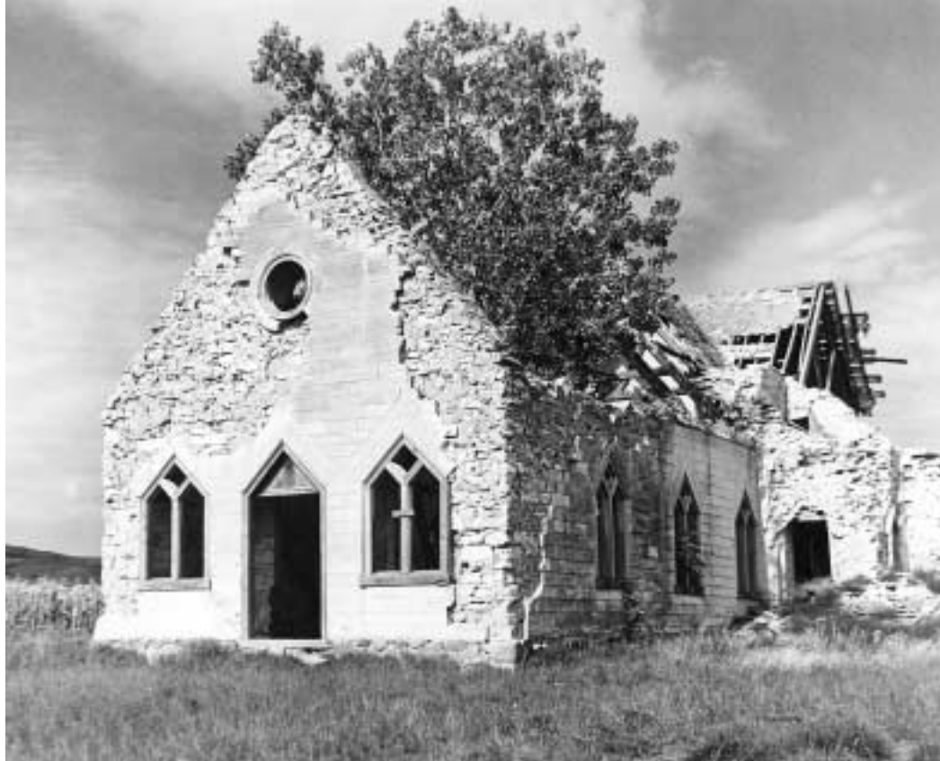
Soldiers at Fort Randall mined chalk rock from quarries about 2 miles south of the fort for their chapel. The 2½-foot blocks were cut by a circular saw run by an old government mule on a treadmill. The bell tower also served as a watch tower. Al Moxon from SDSU later analyzed the stones, finding they contained 20 ppm selenium.
