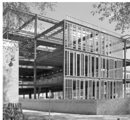
By April the floors were in place and the exterior walls were starting to be erected.
