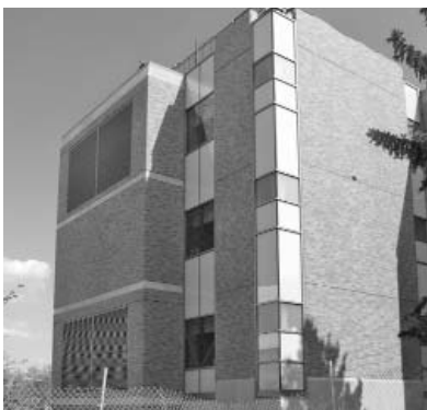
The exterior of the north addition is complete.
