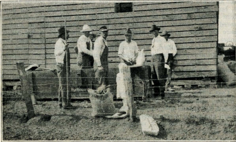
FIGURE 2.—Mixing poisoned bran mash in an ordinary tight wagon box.—Original.
