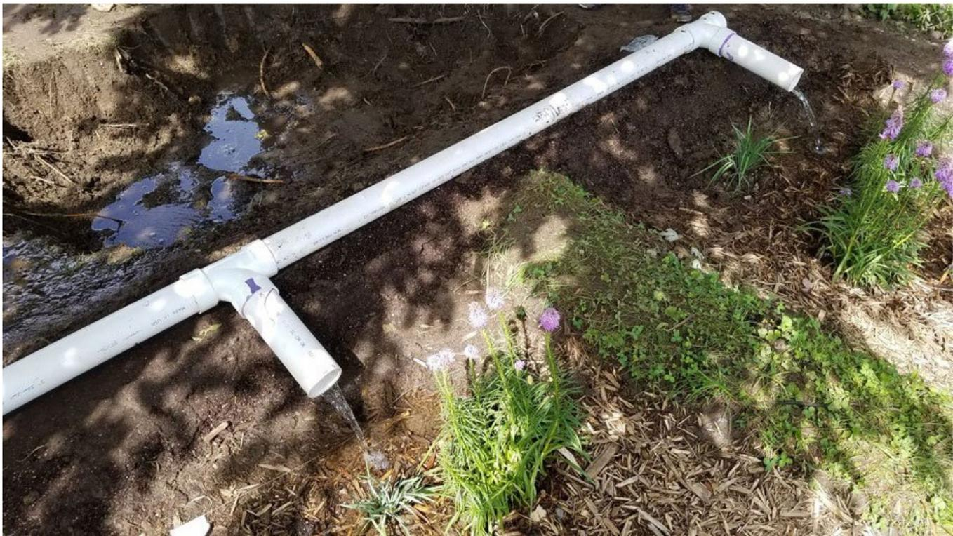
*Water from the downspouts drains through the PVC pipe into the two troughs of the rain garden.*
