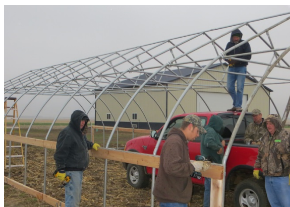
Construction of High Tunnel
