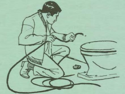
Sometimes objects like toys, pencils or sanitary napkins get in the toilet by mistake. In this case the plunger may not be of much help. Make a hook on the end of a wire. Poke the wire with the hook into the stool and try to pull out the object.
