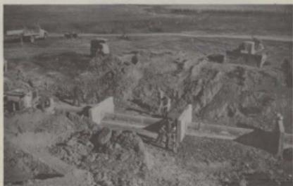
Developing watersheds involves various types of earth moving and dam construction. Here, men are laying the outlet tube for one of the detention dams in the Pattee Watershed in Lincoln County. The tube will run through the base of the completed dam, and will allow the orderly flow of reservoir water to the creek channel below the dam.
