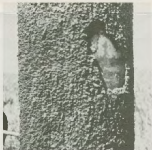
Figure 3. This incrustation was caused by iron bacteria in the water. The jelly-like colloidal substance fills the screen openings and formation voids; it turns hard when exposed to air.
