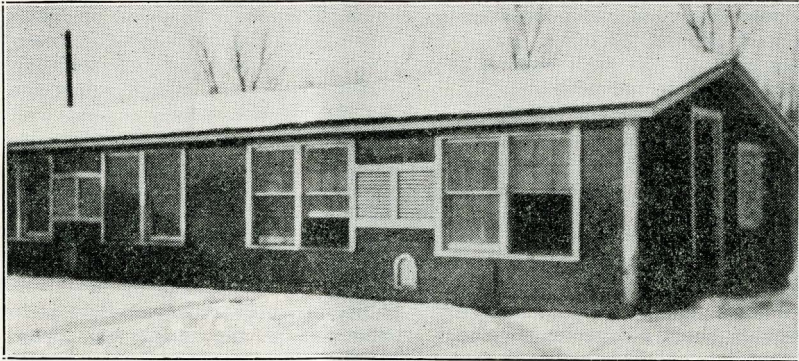
Fig. 19—A REMODELED POULTRY HOUSE
