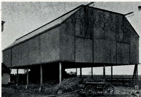
Fig. 50. Typical use of galvanized metal coated with 2 ounces of zinc per square foot. If metal with less coating is used and rusting occurs, brighten rust spots with a wire brush and paint metal with red lead or other good metal paint.
