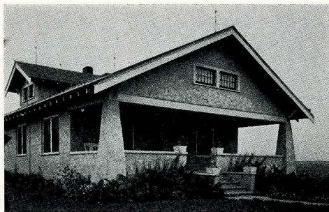
Fig. 53. Stucco houses should be water-proofed to prevent entrance of moisture in walls. (See mixing formulas, page 44.)
