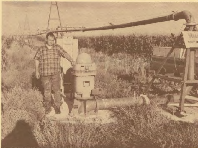
Electric powered irrigation pumps are used on over twice as many acres as diesels. Each electrical power supplier has its own peculiar characteristics you must know.
