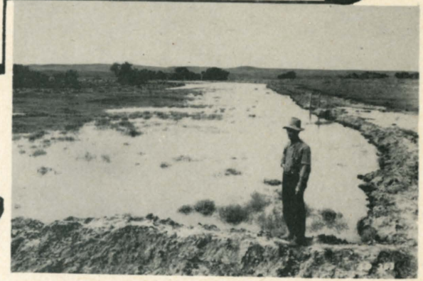
A dike to lead the water
