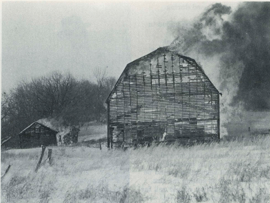
Fig 32. Burning unwanted buildings is best done when the ground has a full cover of snow.
