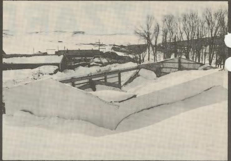
Machine shed roof that heavy, wet snow collapsed in March 1966 blizzard.
