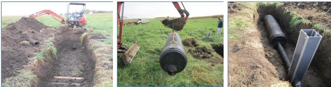
Figure 4.4 Installation of the P adsorption bed control structure near Baltic, South Dakota
