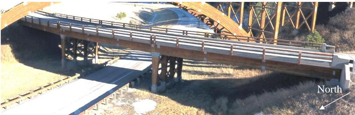
**Fig. 2-2.** Glulam timber girder bridge overview taken by the drone (taken by Luis Duque).
