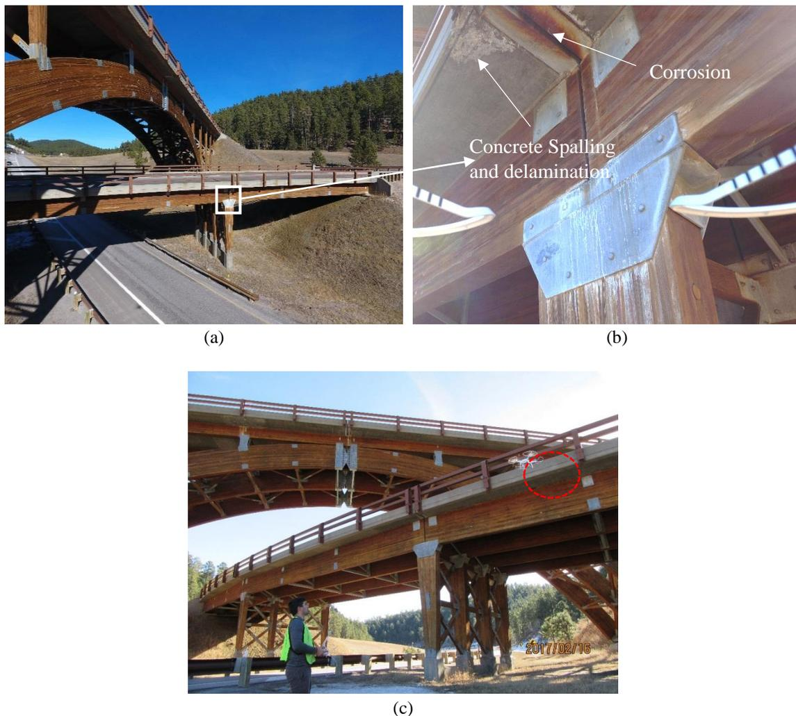
**Fig. 2-7.** Sample images obtained from the timber girder bridge inspection: (a) glulam girder bridge overview (taken by Junwon Seo using drone); (b) damage on timber girder bridge (taken by Luis Duque using drone); and (c) drone flying near girder (taken by Junwon Seo using digital camera).
