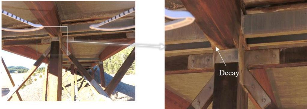
**Fig. 4-6.** Damage identified on Stringer 2 at Joint 4 captured using UAV (taken by Luis Duque using UAV).
