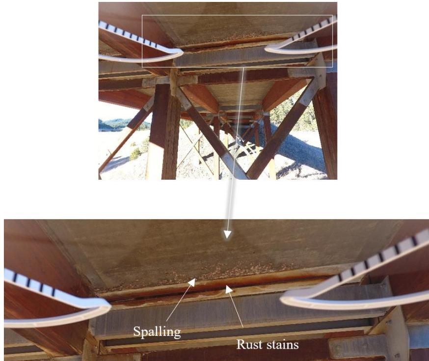
**Fig. 4-5.** Sample damage on Joint 4 captured with UAV (taken by Junwon Seo using UAV).
