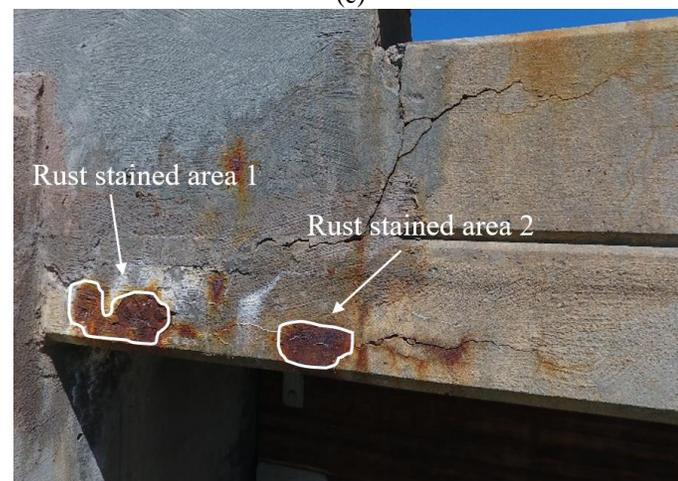
**Fig. 3-9.** Pixel-based damage quantification of damage near abutment of the Keystone Wye Bridge: (a) image aligned with damage; (b) image to the side of damage; (c) identified rust stained areas for image aligned to damage; and (d) identified rust stained areas for the image to the side of damage.
