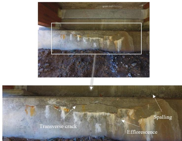
**Fig. 4-7.** Sample abutment damage detected using UAV on Bay 1 at North Abutment (taken by Luis Duque using UAV).
