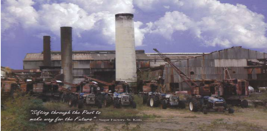
Figure 6. St. Kitts Sugar Factory After Closure. St. Kitts, Circa 2000s, Unknown Photographer (Old Liamuiga & Oualie In Photographs, 2017).
