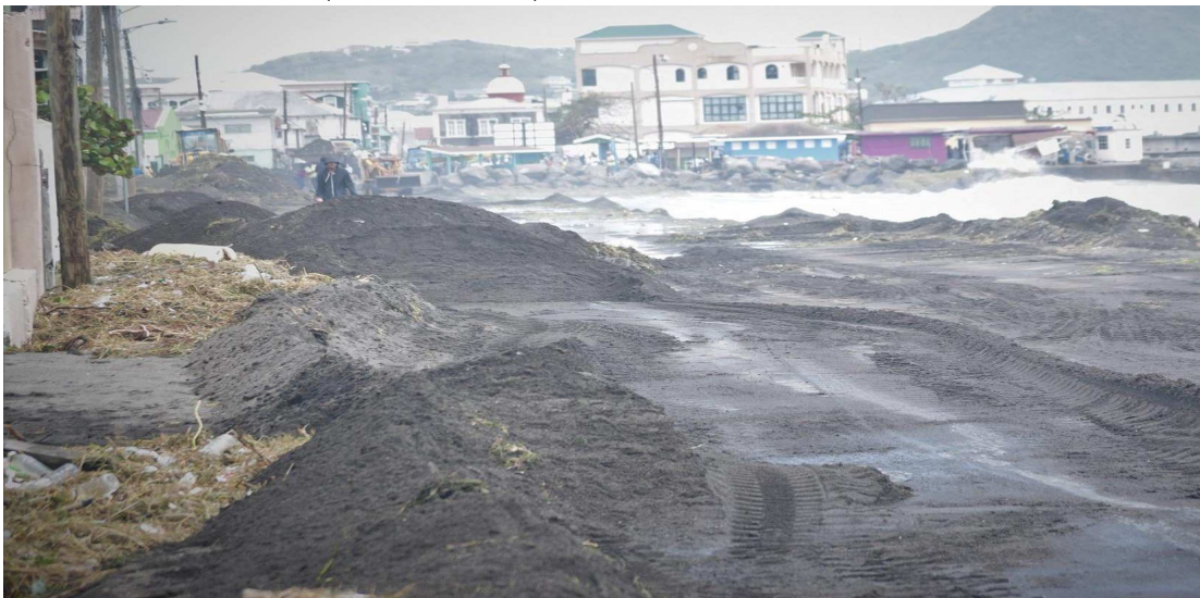
Figure 14. Sand and Wave Change 3. The view of the erosion of Irish Town Bay Road and the St. Kitts Ferry Terminal by waves and sand from Irish Town Bay after hurricane Maria. Unknown Photographer (Mcknight Organization, 2017).
