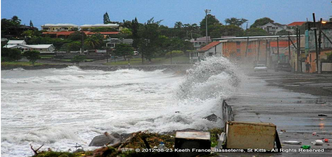
Figure 13. Sand and Wave Change 2. The view of the patterns and size of waves after the construction of man-made piers at West Irish Town Bay and Fort Thomas Road on a windy rainy day. The waves and sand spill over onto the sidewalk and the Street (France 2012).
