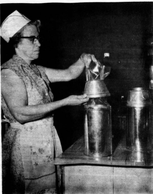
Fig. 2. Drawing bag through holder being placed over receptacle.
