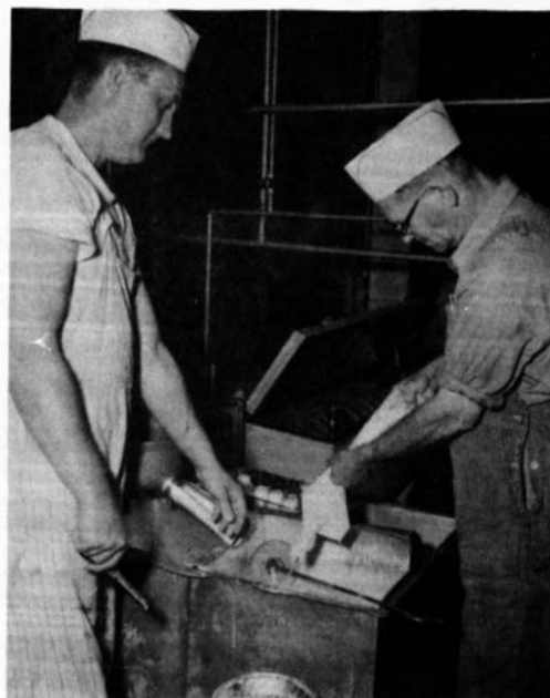
Fig. 9. Stripping cream by hand from bag.
