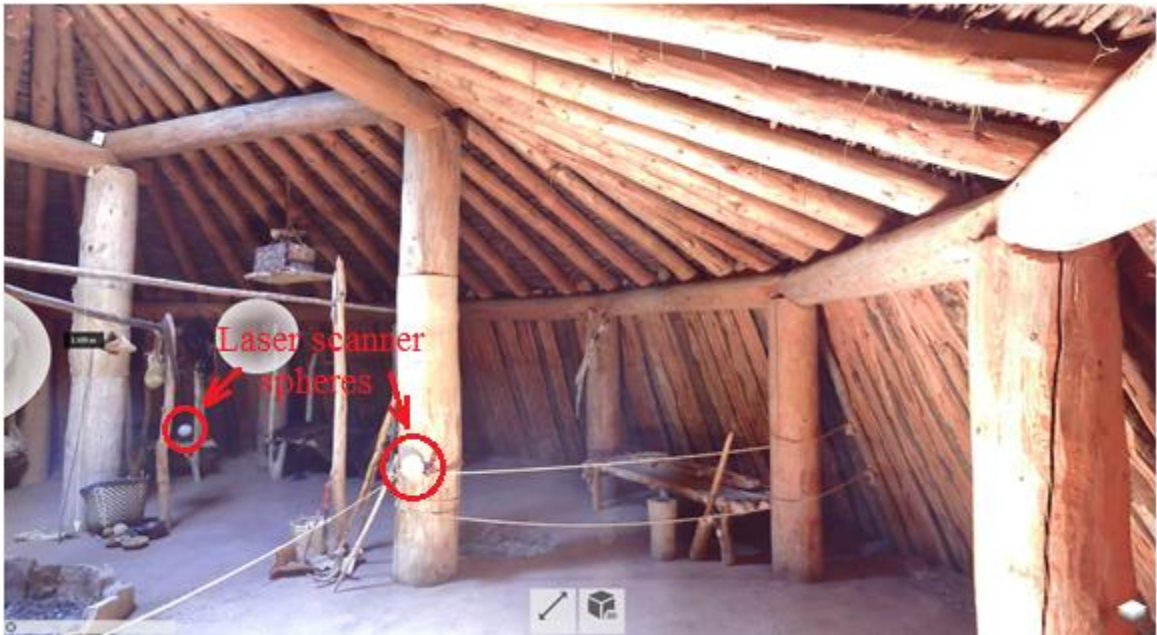
Figure C-10. Autodesk Recap rendering of interior of reproduction earth lodge at the Knife River site showing detail of the short columns and placement of laser scanner spheres (red circles).
