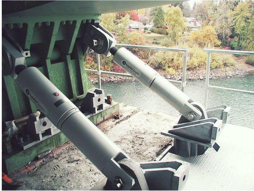
**Figure 3.11 – Seismic damper produced by Taylor Devices Inc. (2019)**
