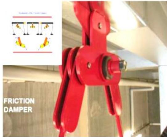
**Figure 3.7 – Rotational friction damper (Heysami, 2015)**
