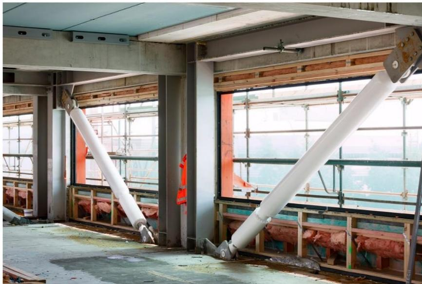
**Figure 3.13 – Viscous damper produced by Victor Seismic (2019)**
