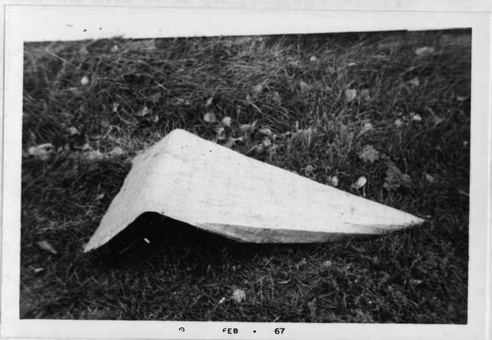
Figure IX. View Illustrating Slope at Rear of Row Crop Unit
