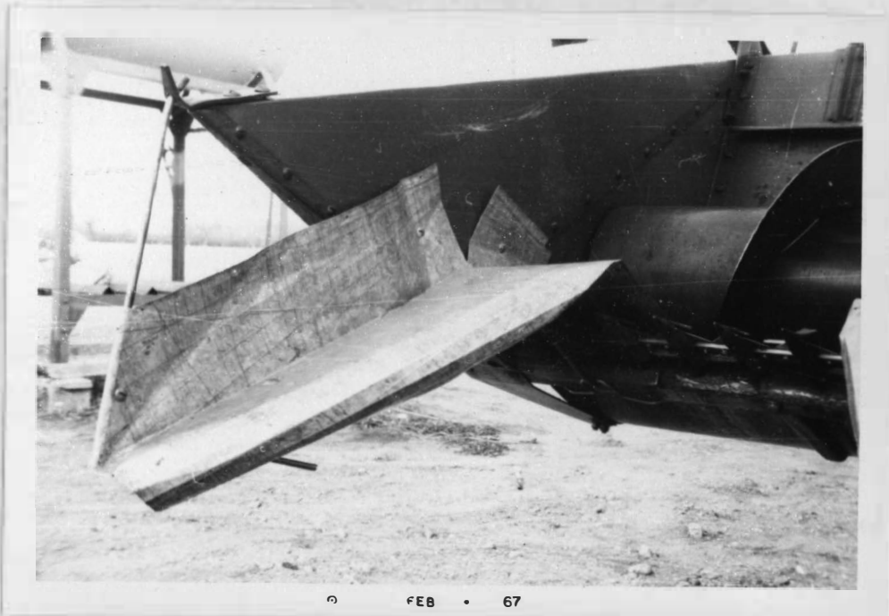
Figure X. Row Crop End Snout in Position on Machine
