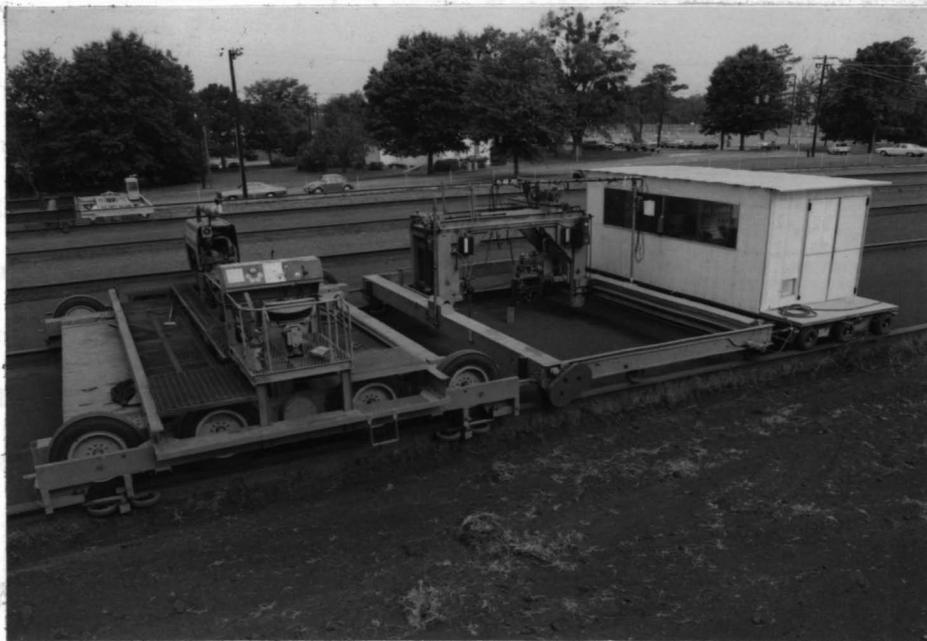
Figure 5. Arrangement of the power, dynamometer, and instrument cars
