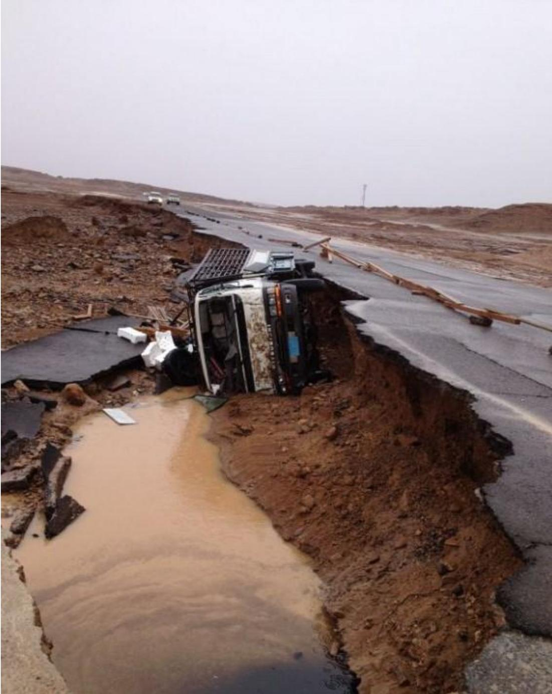
Figure 4.15 Road collapse and one vehicle was sent off the road after intense rainstorm (01/18/2010).
